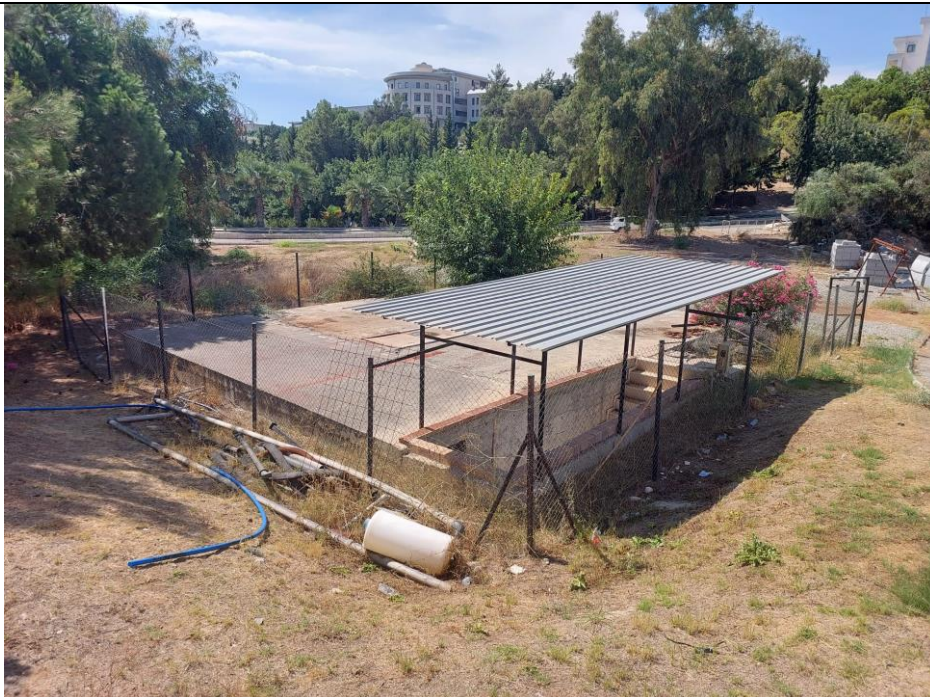
Rainwater Harvesting System
