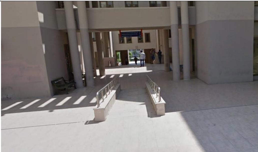
Mersin University disabled ramp
