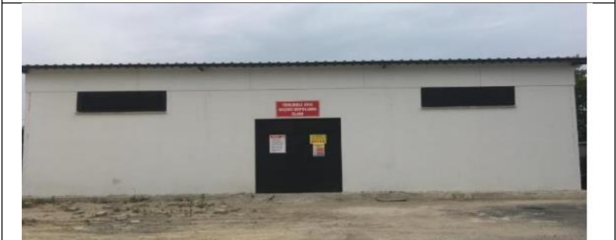
Example of Inorganic Waste Treatment (Mersin University, Turkey)
