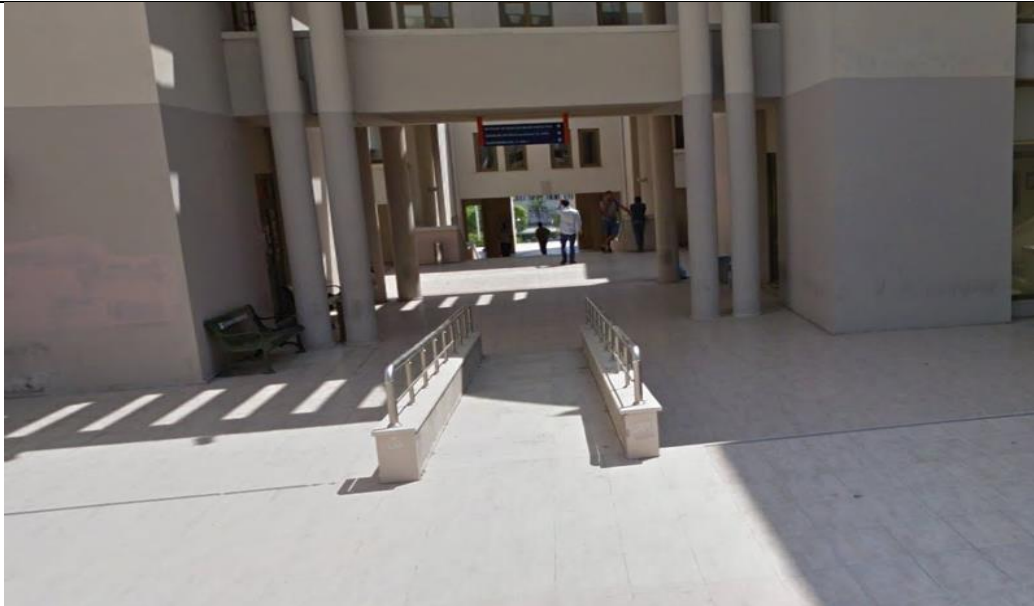
Mersin University disabled ramp
