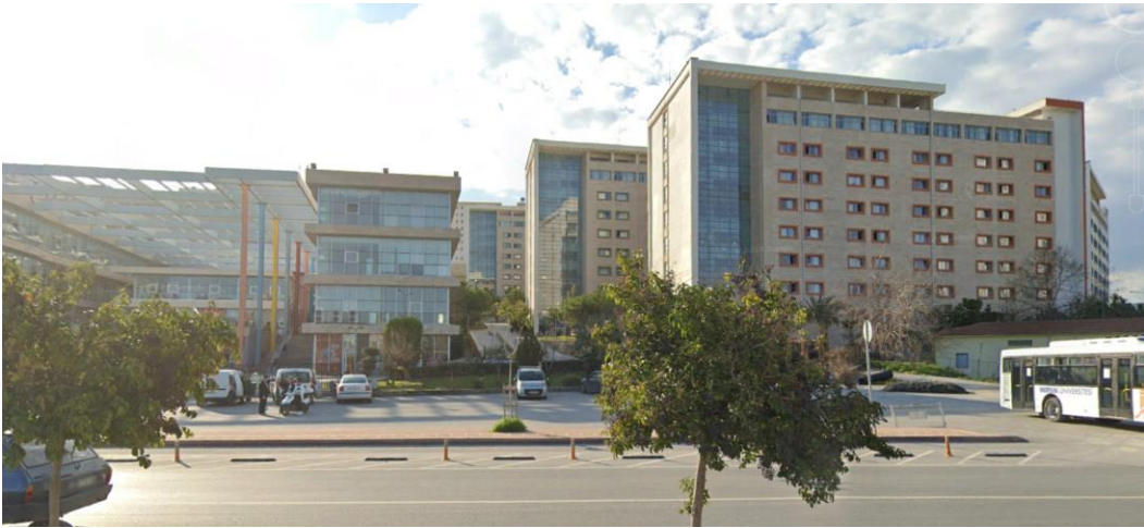
Some of the dormitory buildings where grey water application is applied
