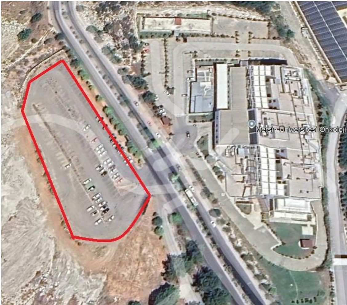
A new car parking area will be opened opposite the Oncology Hospital and will be covered and solar energy panels will be installed to save energy.
