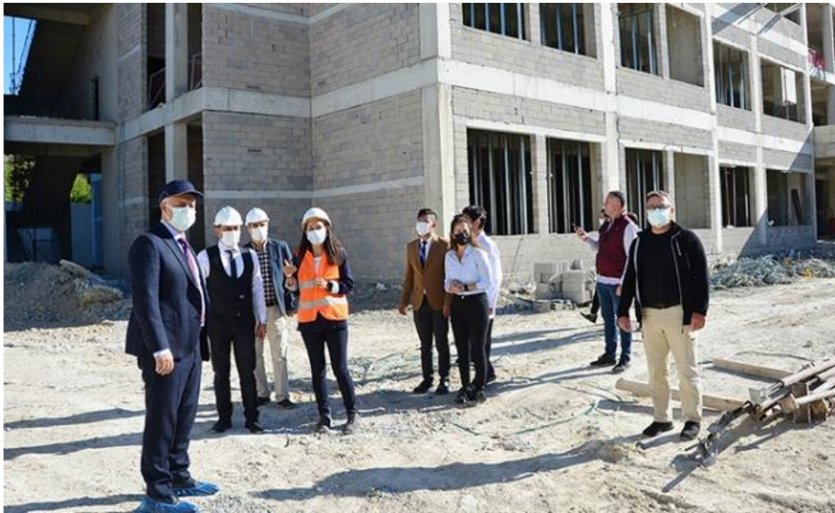
Construction of Mersin University Dental Hospital is underway.
