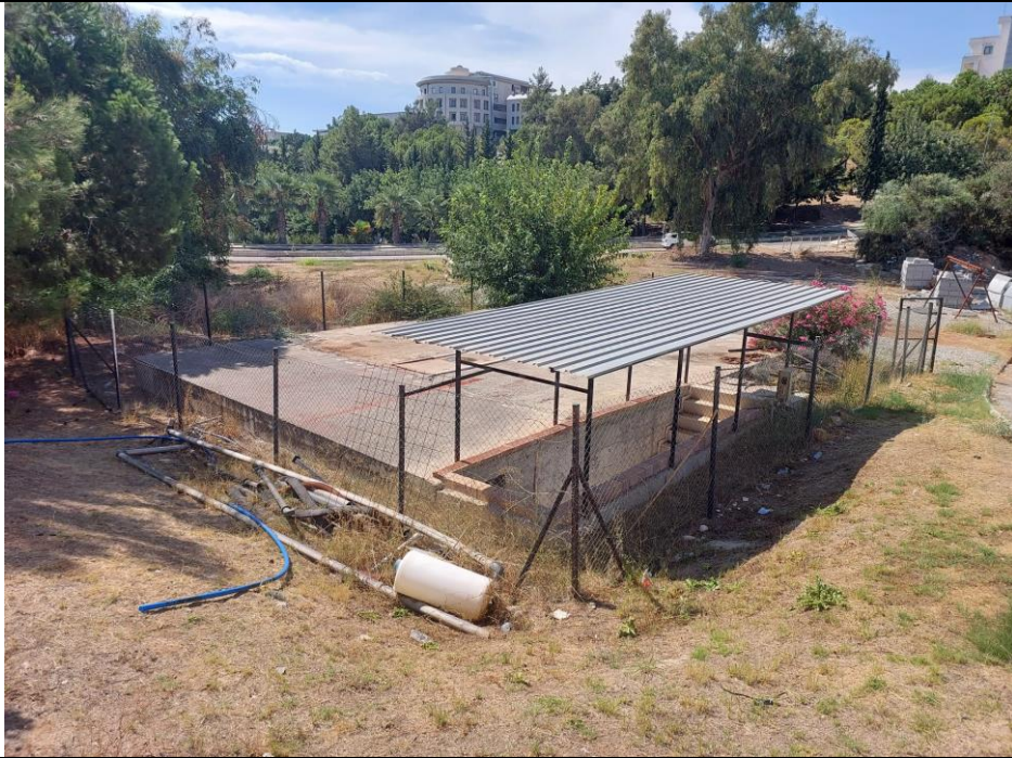
Rainwater Harvesting System
