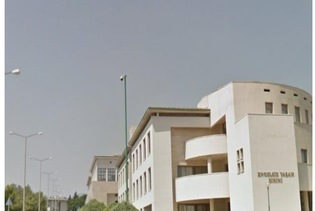
CCTV in all buildings
