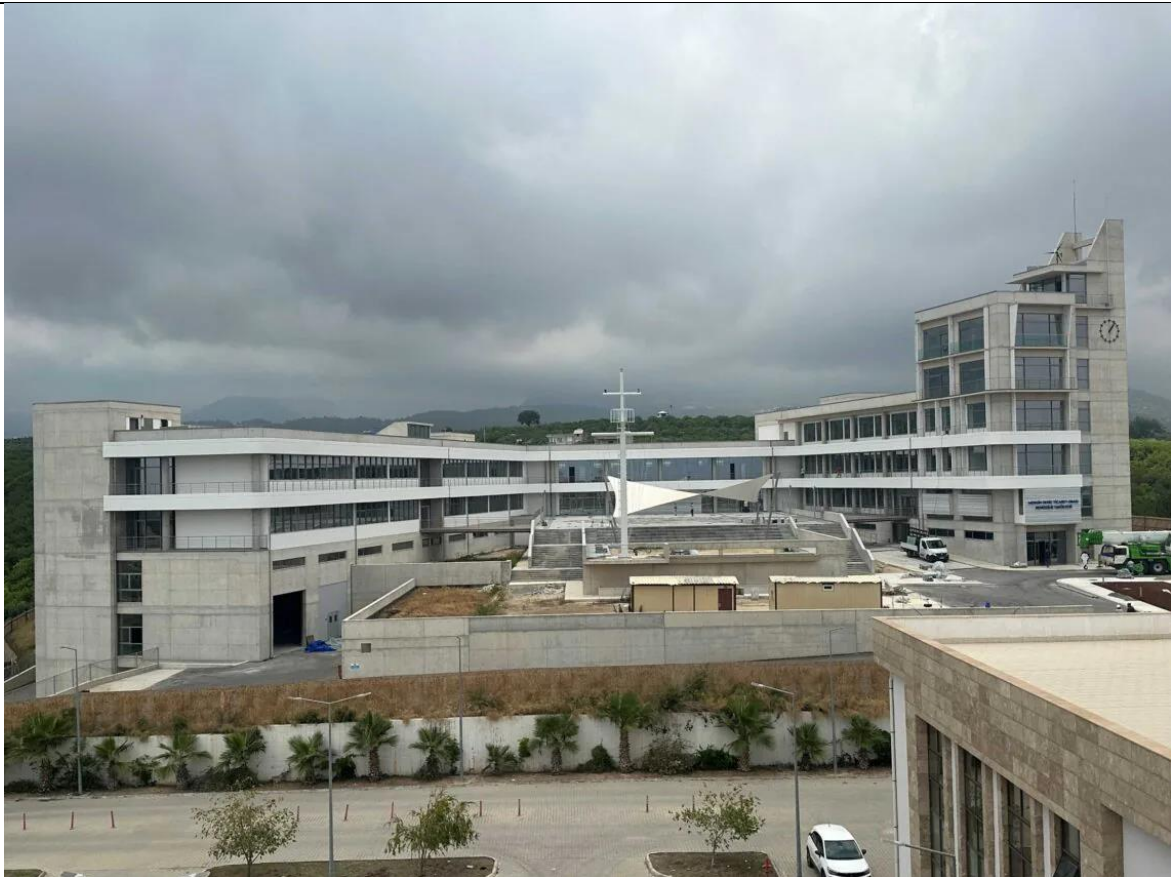
Mersin University Maritime Faculty Construction
