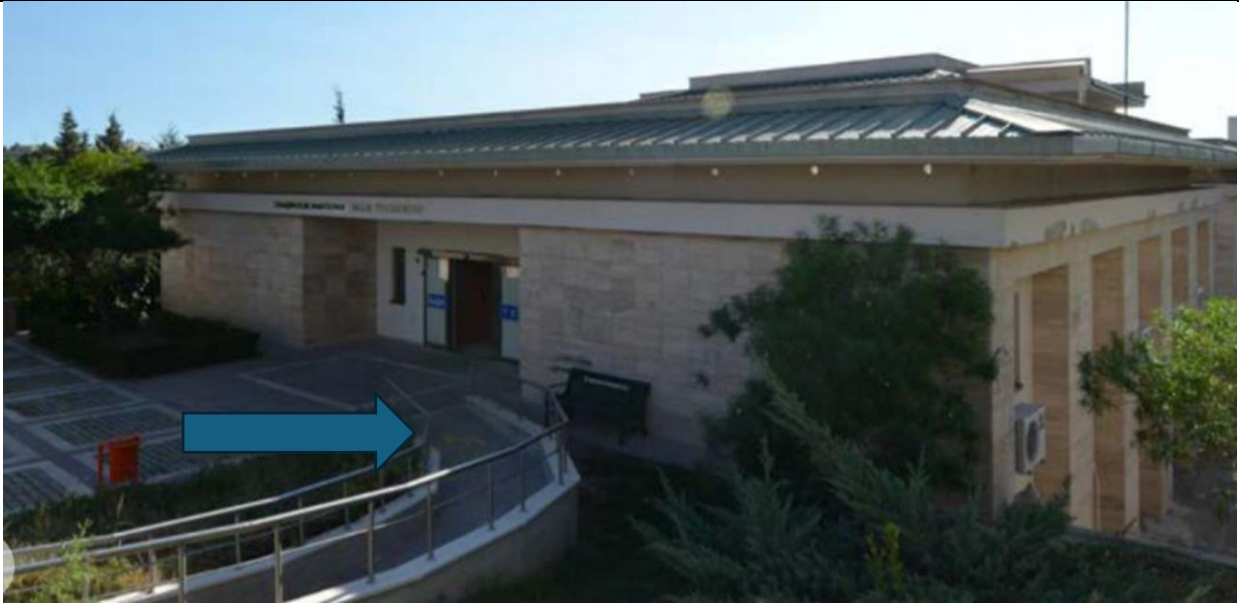
Mersin University disabled ramp
