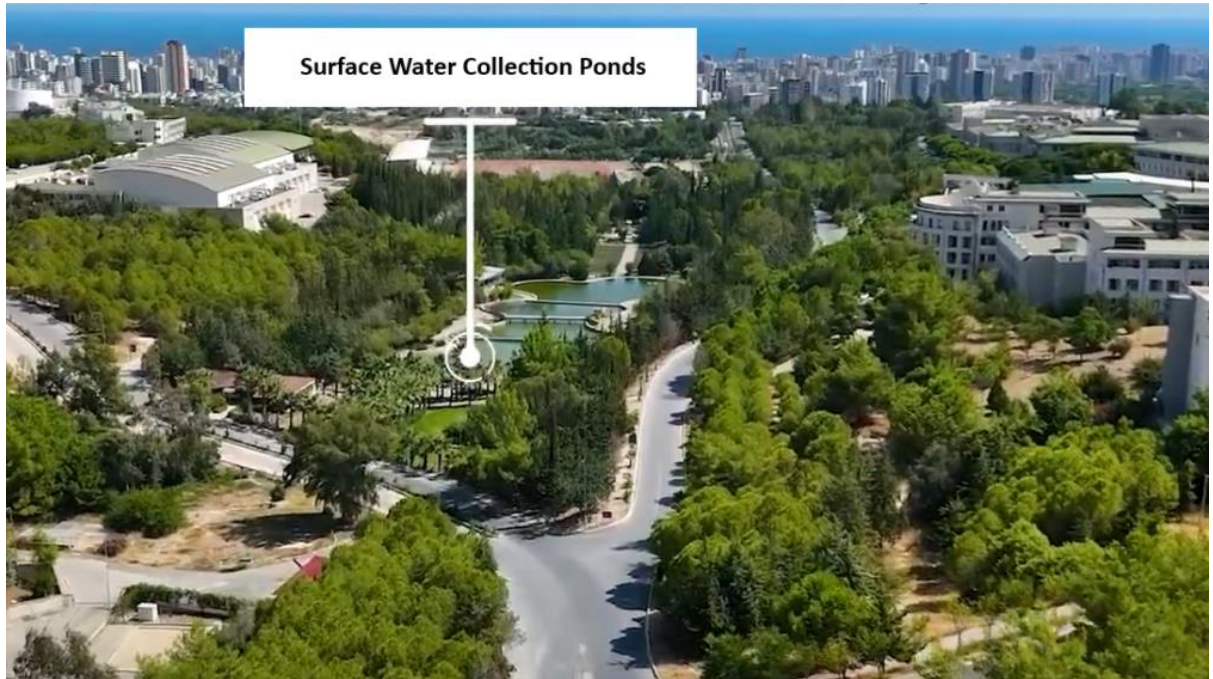
Surface Water Collection Ponds
